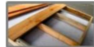
Middle ribs should be 12" from the end.
