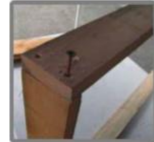
Pilot holes prevent the wood from cracking.
